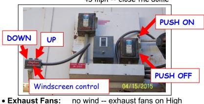
no wind -- exhaust fans on High < 15 mph -- exhaust fans on low > 20 mph -- exhaust fans OFF
